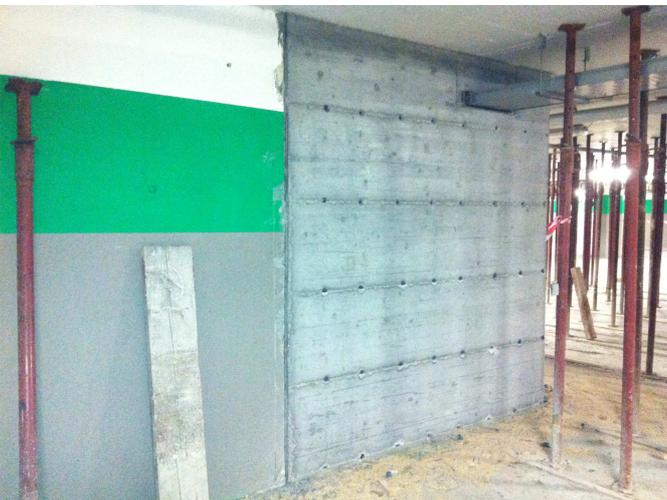
Figure 8. Strengthening existing bracing elements / Controventi esistenti irrobustiti
